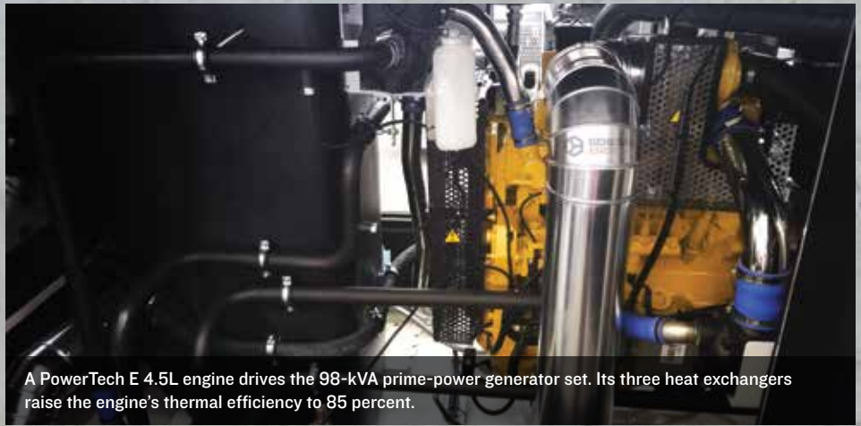
The engines' configurations enabled Genesal to adapt the design of the CHP multi-energy system to peak efficiency. Should the micro-network fail, the two groups of generators change their mode of operation to ensure a constant flow of energy.
