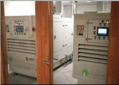
The engines' configurations enabled Genesal to adapt the design of the CHP multi-energy system to peak efficiency. Should the micro-network fail, the two groups of generators change their mode of operation to ensure a constant flow of energy.
