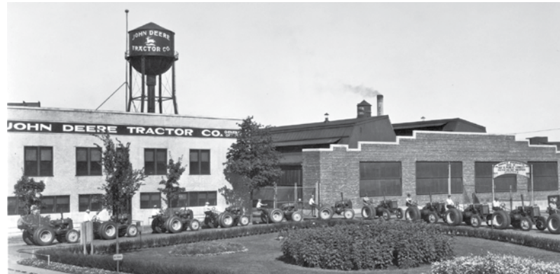
Top: Model "D" tractors take shape on the Waterloo Works assembly line in 1924. Above: The 1931 Model "D" line outside of John Deere Waterloo Works.
