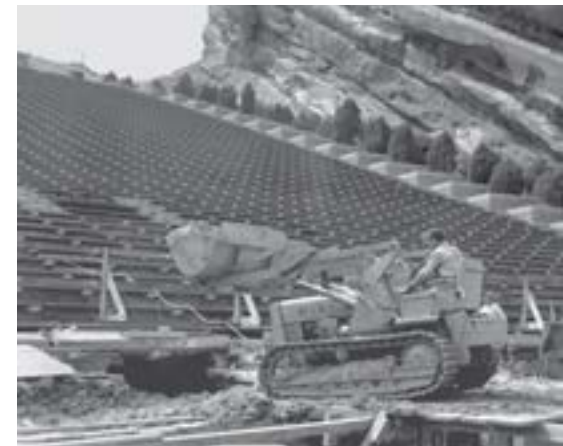
A 440C Crawler outfitted with an 831 Loader is shown here busy at work in 1959 on the construction of the Red Rocks Amphitheatre in Denver, Colorado.
